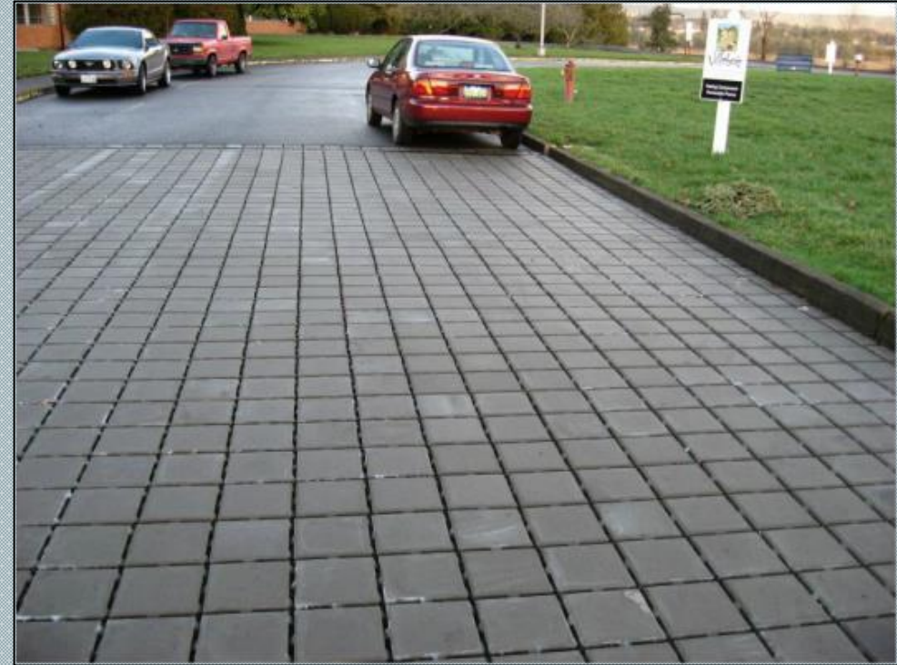
Permeable Paving
