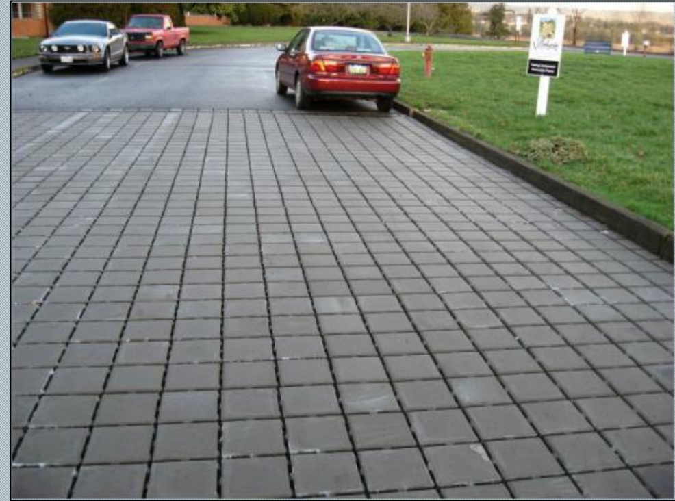
Permeable Paving
