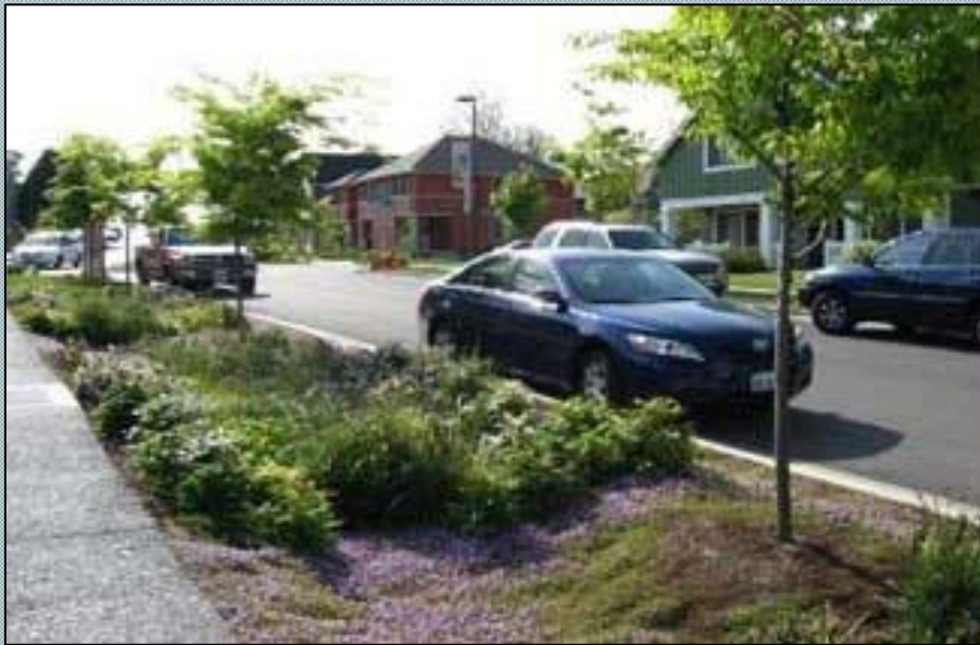
Bioswale between sidewalk and street
